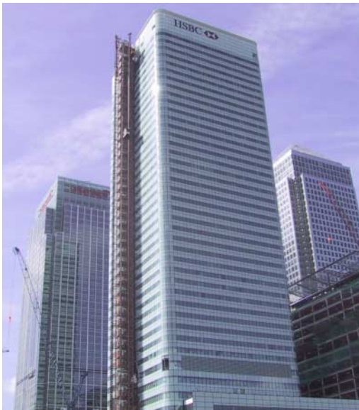
The HSBC Group Headquarters building under construction in the United Kingdom
