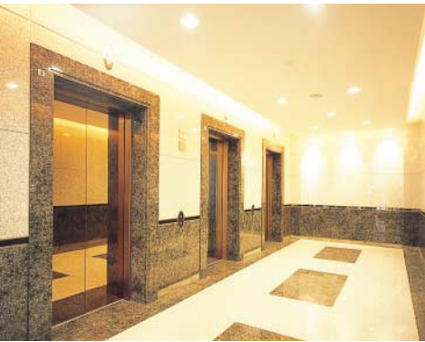
Elevators installed at the Keppel Bank Headquarters building in Singapore
