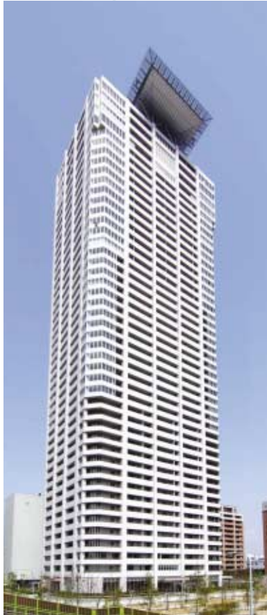
Mid Capital Tower
