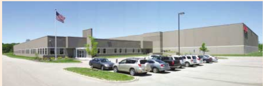
Fujitec America's New Head Office and Plant
