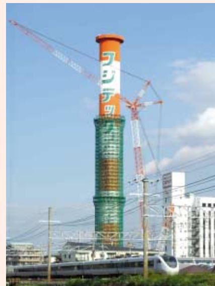
Elevator research tower currently being disassembled (Ibaraki)
