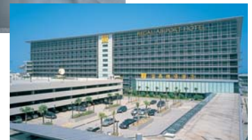
Fujitec moving walkways operating at Regal Airport Hotel in Hong Kong
