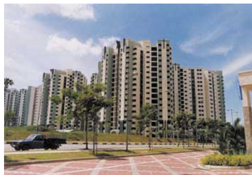
HDB high-rise residential buildings
