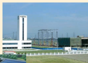
Construction site where work is progressing at a quick pace
