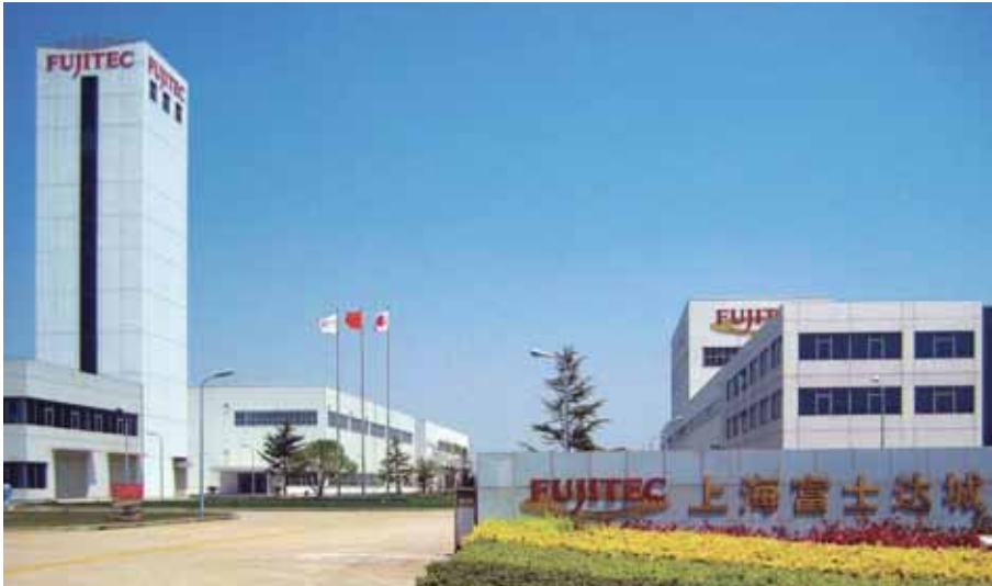
Shanghai Fujitec City (from left, Fujitec Shanghai Technologies Co, Ltd., Fujitec Shanghai Sourcing Center Co., Ltd., and Shanghai Huasheng Fujitec Escalator Co., Ltd.)
