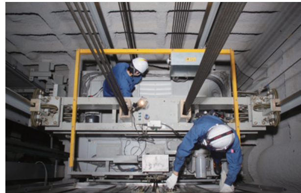
Elevator maintenance operations
